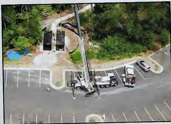
Cranes place the shipping containers in place. The reinforced-steel containers will serve as the base structure for the new classroom, but will not be visible in the completed design. (Design rendering at right.)
